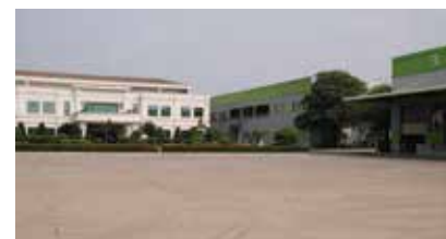
The office building and some factory halls at DDK Group's factory in Vietnam.
